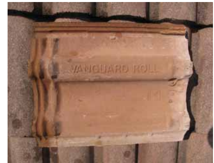
Figure 4: Bottom surface of a concrete Vanguard Roll roof tile with imprints of the style name and the Monier Lifetile (box with ML) manufacturer mark
