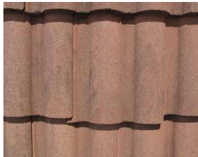
Figure 3: Top surface of a concrete Vanguard Roll roof tile manufactured by Monier Lifetile
