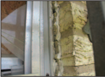
Figure 11: Displaced window frame and fractured glazing
