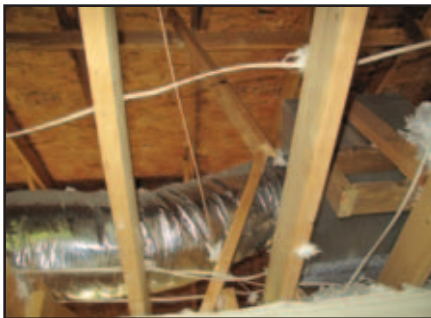
Figure 5: Vertical strut fractured in compression
