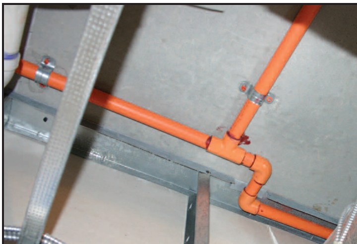
Figure 1. CPVC pipe installation in a fire protection system.
