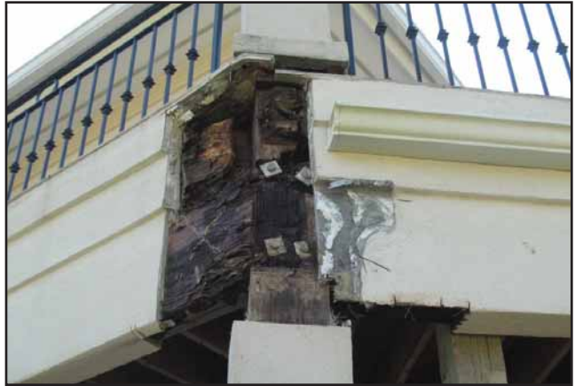
Figure 1: Exposed balcony assembly
